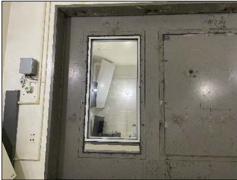
Photo No. 1 Interior View of Installed Test Specimen
